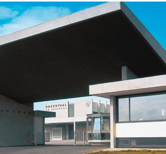
Rosenthal am Rothbühl factory, designed by W. Gropius
